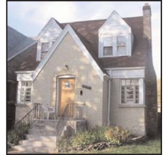
This Berwyn home received a complete weatherization assessment, including safety inspections of the fireplace and furnace.
