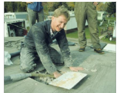
Figure 41612-1: Blowing insulation through mobile home roof
