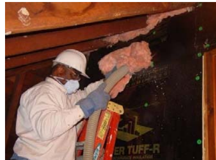
Figure 21364-3: Knee walls being dense-packed with cellulose
