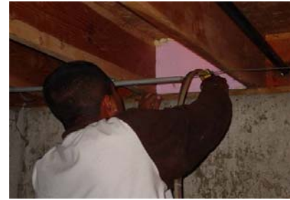
Figure 2172-1: Rigid foam board sealed in place with 2-part spray foam
