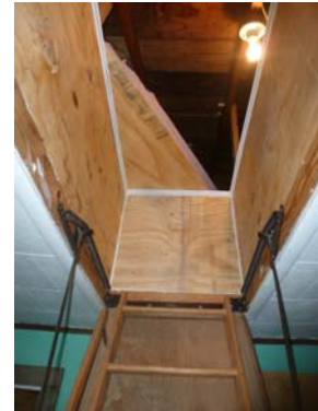
Figure 2135-2: Box around retractable attic stairs
