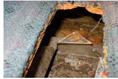
Figure 4114-1: Opening between duct boot and floor
