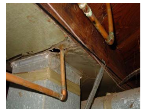
Figure 31531-5: Seal holes in ducts
