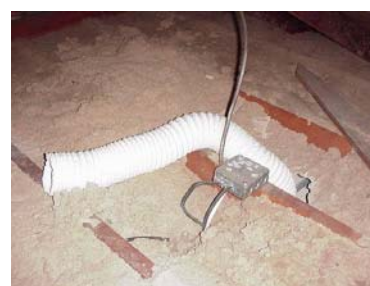
Figure 507-1: Fans may not be vented into the attic under the Weatherization Program
