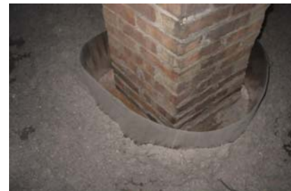
Figure 2131-3: Metal barrier around chimney
