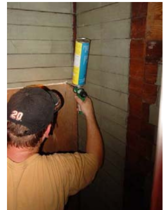
Figure 21232-1: 1-part spray foam; foam canister is screwed onto a foam gun
