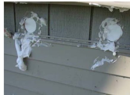
Figure 2144-3: Holes sealed with foam plugs
