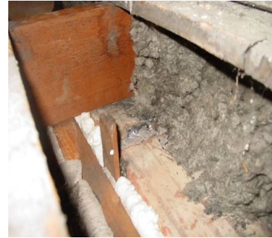
Figure 2122-6: Fur cavity sealed with 2-part spray foam
