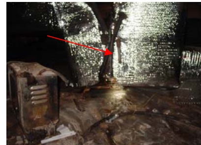
Figure 2154-2: Condensate line draining on top of ground moisture barrier
