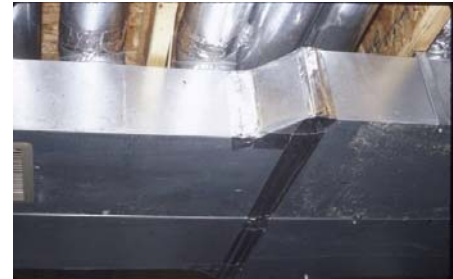
Figure 3124-1: Repair duct system
