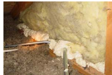
Figure 2122-3: Stud cavity sealed with 2-part spray foam
