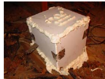
Figure 2131-1: Recessed light covered with drywall box
