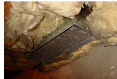
Figure 3114-2: Dirty combustion air intake to wood stove that needs to be cleaned
