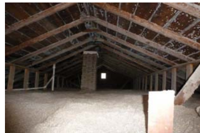
Figure 2122-8: Cut-off chimney in attic
