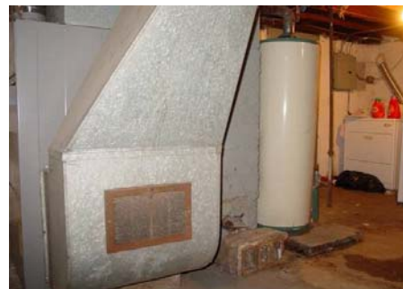
Figure 31531-6: Return air grilles should be sealed
