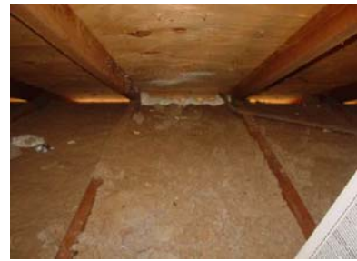
Figure 2122-13: Exterior wall top plate under low-pitch roof sealed with foam gun shown in Figure 2122-10.
