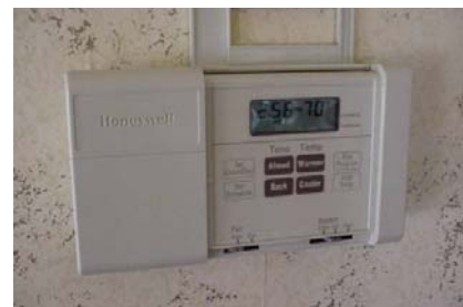
Figure 318-2: Automatic setback thermostat
