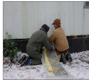
Figure 41521-1: Batt-stuffing a mobile home wall
