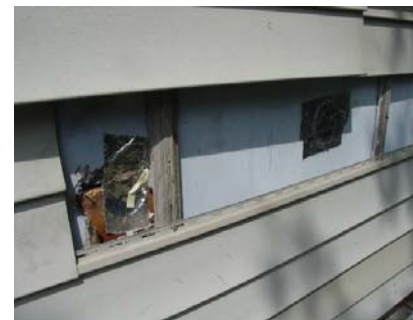
Figure 2142-2: Hole sealed with sheathing tape
