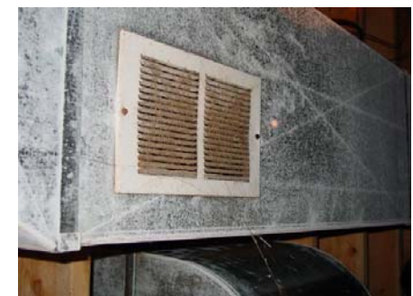
Figure 31531-4: Permanently seal registers in unconditioned spaces
