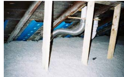
Figure 21324-2: Soffit chutes extended above insulation
