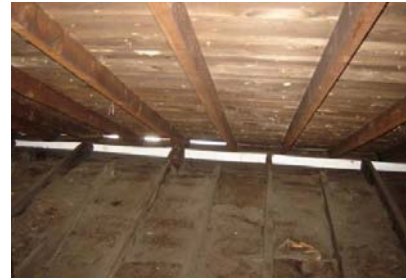
Figure 21324-1: Foam blocking installed over top plates
