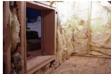
Figure 21364-1: Knee walls insulated with fiberglass insulation
