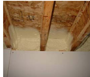
Figure 2171-1: 2-part spray foam on rim joist
