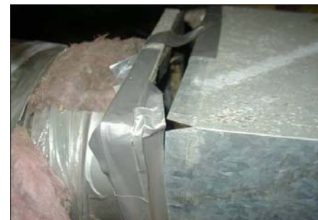
Figure 31532-3: Tape is not expected to hold a joint together
