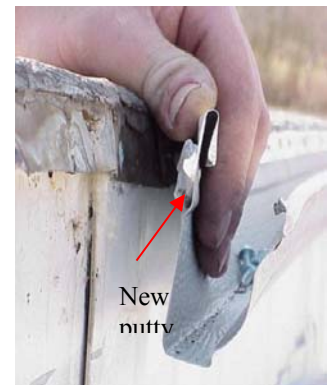
Figure 41611-3: Re-installing roof gutter with new putty tape
