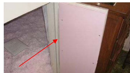
Figure 21365-1: Knee wall hatch insulated and weatherstripped
