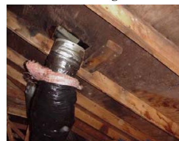
Figure 507-2: Venting to a roof vent is not allowed under the Weatherization Program; a roof vent may be removed and the exhaust duct extended through the existing hole and capped with a termination kit
