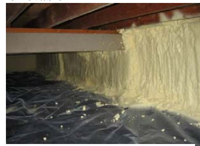
Figure 2154-1: Minimum 6 mil ground cover; sealed to foundation wall with 2-part foam
