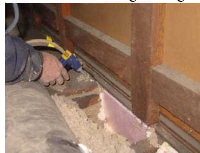
Figure 2122-1: Sealing joist cavity under knee wall with foam board and 2-part spray foam
