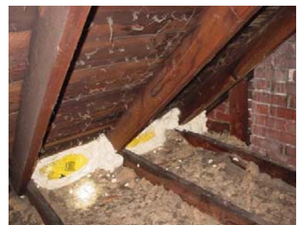
Figure 2122-5: Balloon framed stud cavity sealed with fiberglass batts stuffed in cellulose insulation bags
