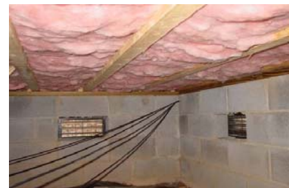
Figure 2152-1: Insulation should fill floor cavity
