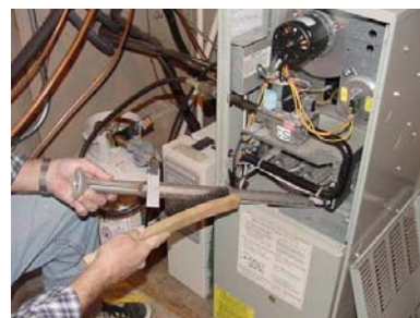
Figure 31111-2: Clean burners with stiff brush
