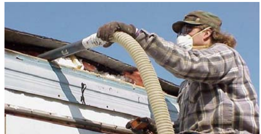
Figure 41611-2: Blowing roof cavity from edge
