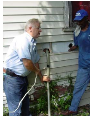
Figure 2142-1: Dense-pack cellulose being installed
