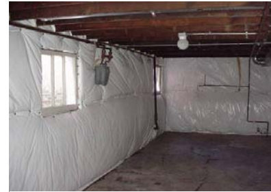
Figure 2162-1: Vinyl faced fiberglass insulation
