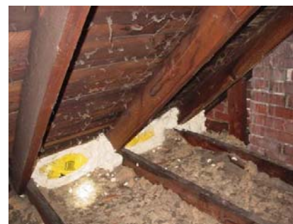
Figure 2122-5: Balloon framed stud cavity sealed with fiberglass batts stuffed in cellulose insulation bags
