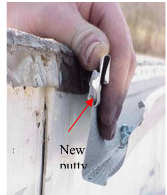
Figure 41611-3: Re-installing roof gutter with new putty tape
