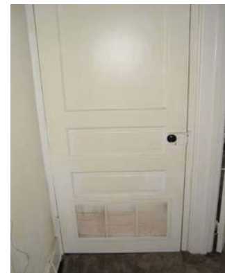
Figure 3124-3: Transfer grille
