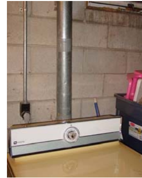
Figure 508-1: Dryers should be vented with smooth metal duct
