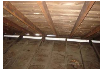
Figure 21324-1: Foam blocking installed over top plates
