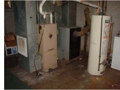
Figure 312-2: Combustion appliance zone: note presence of grille in return air duct that can cause depressurization of the water heater
