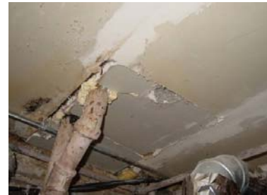
Figure 2122-11: Cavity beneath bathtub sealed with gypsum board and dense-packed with cellulose
