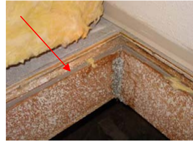
Figure 2153-1: Peel & stick weatherstripping is not permitted
