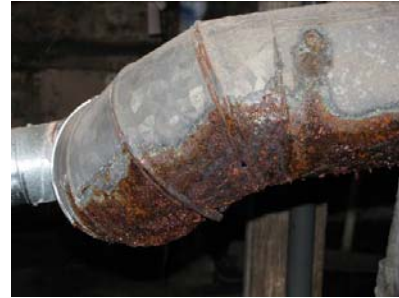
Figure 31111-4: Check vent for condensation problems
