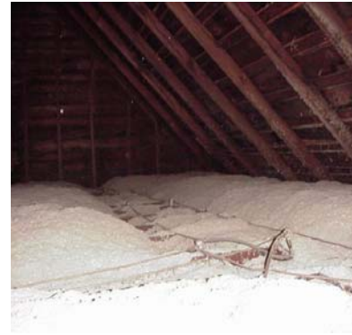
Figure 2131-4: Attic insulation installed under knob-and-tube wiring
