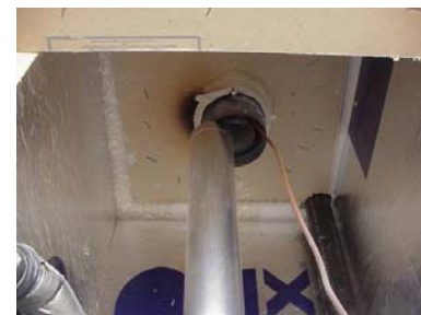
Figure 31111-3: Ensure that vent is properly connected
