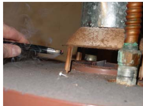
Figure 117-2: Failed spillage test
