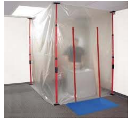
Figure 5136-2: Level 2 Containment
