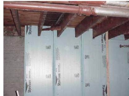
Figure 2161-1: Rigid foam board basement wall insulation
