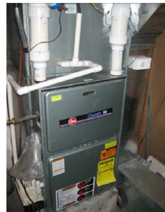
Figure 3133-1: Direct vent sealed combustion furnace
