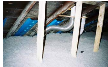
Figure 21324-2: Soffit chutes extended above insulation
