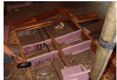
Figure 2131-5: Rigid foam board used as barrier next to K&T wiring; floor cavity will be blown with cellulose insulation
