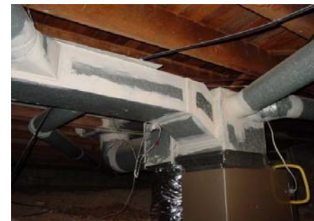
Figure 31532-2: Duct mastic used to seal duct joints
