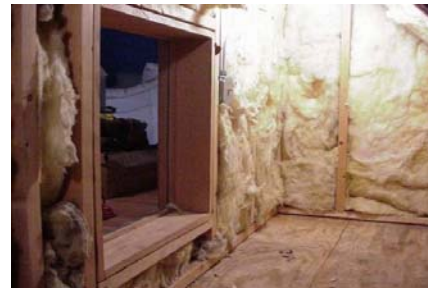
Figure 21364-1: Knee walls insulated with fiberglass insulation
