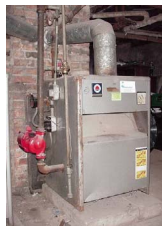
Figure 3161-1: Warm water boiler
