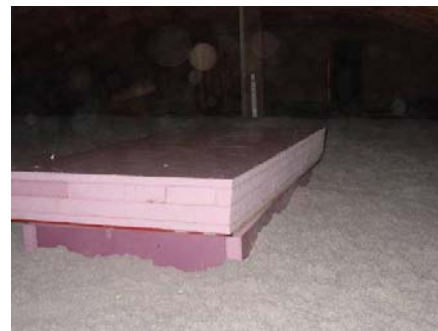
Figure 2135-1: Attic hatch insulated with foam board; plywood blocking has been insulated with foam board
