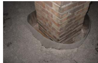
Figure 2131-3: Metal barrier around chimney
