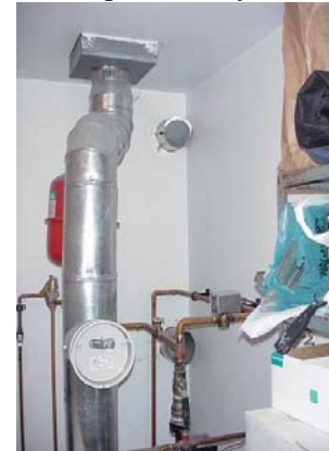
Figure 3124-2: Combustion air intake
