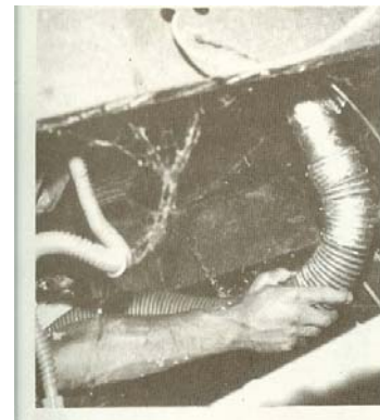
Figure 41422-1: Belly-board method
