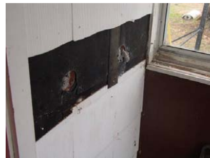
Figure 2141-1: Asbestos siding that has been removed
