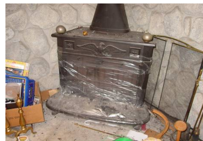
Figure 1111-1: Ensure that ashes are not drawn into the home during the blower door test
