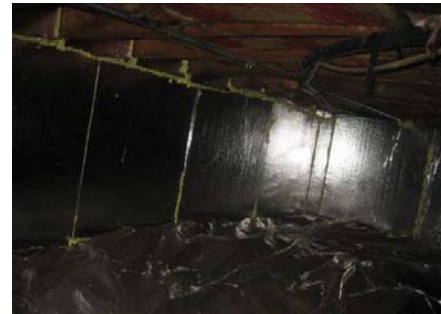
Figure 2151-1: Foil-faced rigid foam board on foundation walls, vents sealed and continuous and sealed
