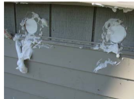
Figure 2144-3: Holes sealed with foam plugs
