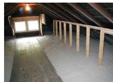
Figure 21332-1: Insulation blown under floor boards and then over floor boards where client storage is not needed
