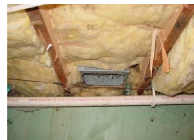
Figure 2151-3: Combustion air intake from crawl space; floor above crawl space is thermal boundary
