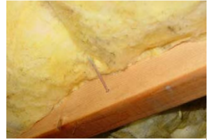
Figure 2152-3: Compressed insulation due to insulation support
