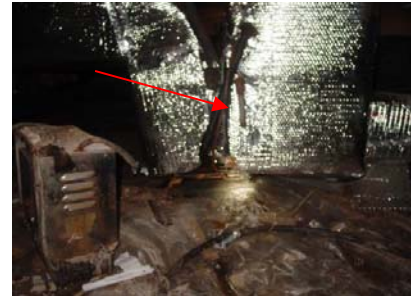
Figure 2154-2: Condensate line draining on top of ground moisture barrier
