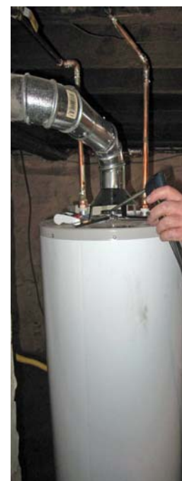
Figure 3123-1: CO reading taken for water before dilution air
