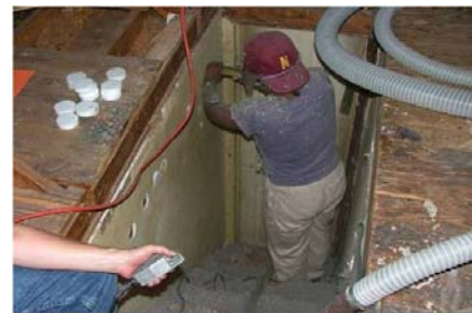
Figure 2135-3: Stairwell walls being dense-packed
