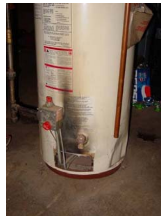
Figure 31111-1: Evidence of flame roll-out
