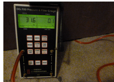
Figure 1152-1: Room to room pressure is 31.6 Pa!
