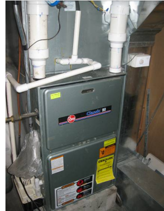
Figure 3133-1: Direct vent sealed combustion furnace
