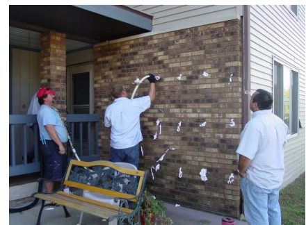
Figure 2144-2: Injection foam used to insulate brick veneer wall
