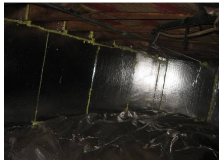
Figure 2151-1: Foil-faced rigid foam board on foundation walls, vents sealed and continuous and sealed
