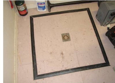
Figure 2153-2: Crawl space access hatch; weatherstripped and easily removable
