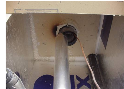
Figure 31111-3: Ensure that vent is properly connected
