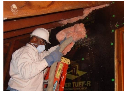
Figure 21364-3: Knee walls being dense-packed with cellulose
