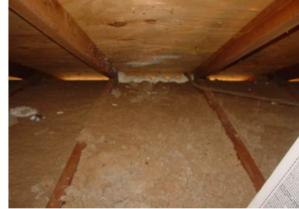
Figure 2122-13: Exterior wall top plate under low-pitch roof sealed with foam gun shown in Figure 2122-10.
