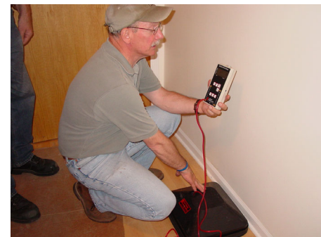
Figure 114-1: Pressure pan test
