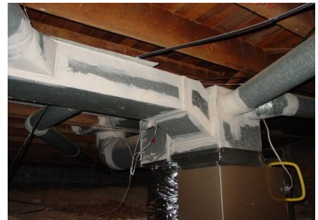
Figure 31532-2: Duct mastic used to seal duct joints
