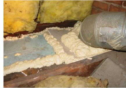
Figure 2122-10: Duct chase sealed with foam board and 2-part spray foam
