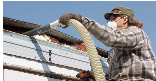
Figure 41611-2: Blowing roof cavity from edge
