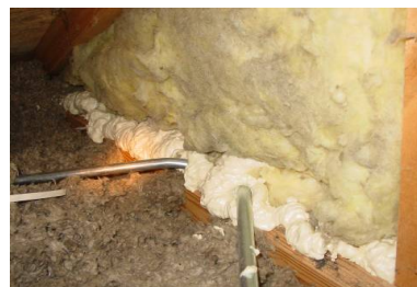
Figure 2122-3: Stud cavity sealed with 2-part spray foam
