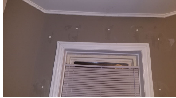
Figure 2144-3: Holes sealed and ready for painting
