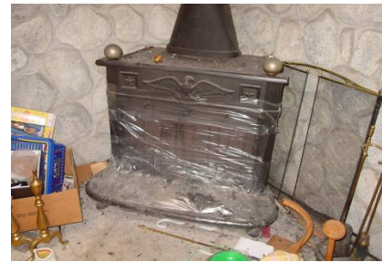
Figure 1111-1: Ensure that ashes are not drawn into the home during the blower door test
