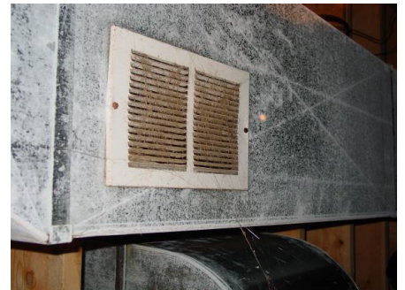
Figure 31531-4: Permanently seal registers in unconditioned spaces
