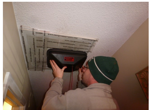
Figure 1141-2: Duct partially covered with duct mask tape.
