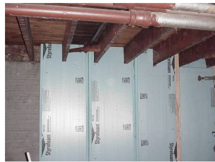
Figure 2161-1: Rigid foam board basement wall insulation
