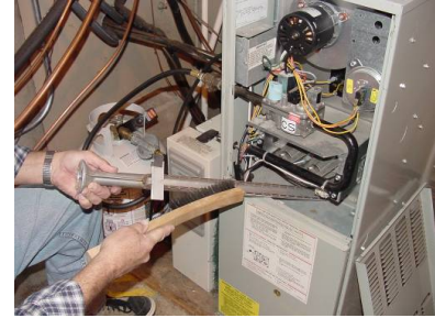
Figure 31111-2: Clean burners with stiff brush
