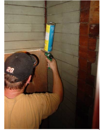
Figure 21242-1: 1-part spray foam; foam canister is screwed onto a foam gun
