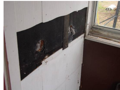
Figure 2141-1: Asbestos siding that has been removed
