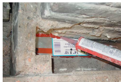
Figure 2122-7: Seal chimney bypass with sheet metal and high temperature sealant
