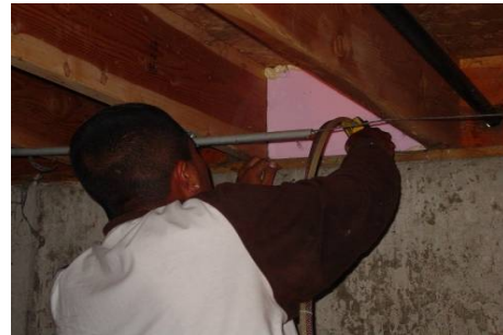
Figure 2172-1: Rigid foam board sealed in place with 2-part spray foam
