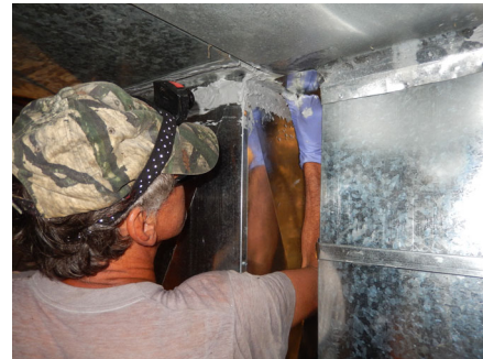
Figure 3124-1: Repair duct system
