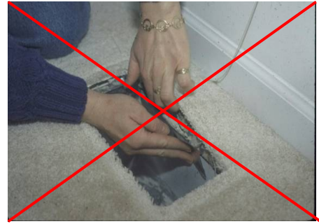
Figure 31532-1: Tape is not to be used for sealing ducts in the Illinois WX Program
