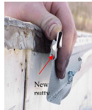
Figure 41611-3: Re-installing roof gutter with new putty tape
