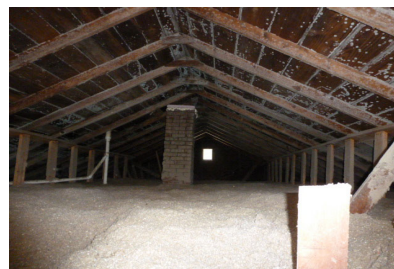
Figure 2122-8: Cut-off chimney in attic
