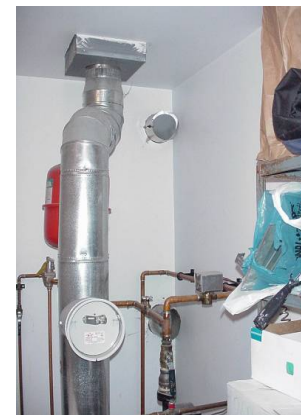
Figure 3124-2: Combustion air intake
