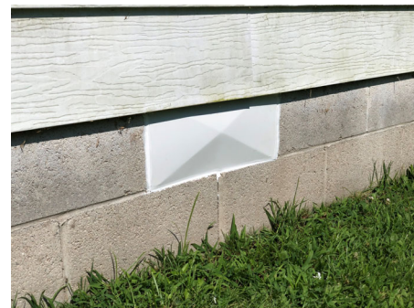
Figure 2155-1: Insulated vent with metal cover.
