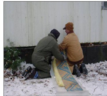
Figure 41521-1: Batt-stuffing a mobile home wall
