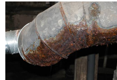
Figure 31111-4: Check vent for condensation problems
