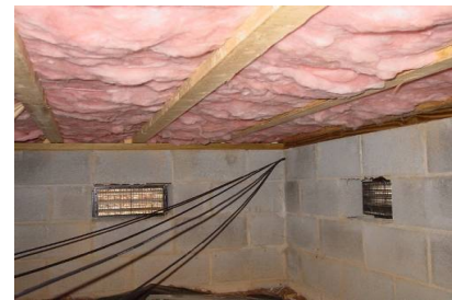
Figure 2152-1: Insulation should fill floor cavity
