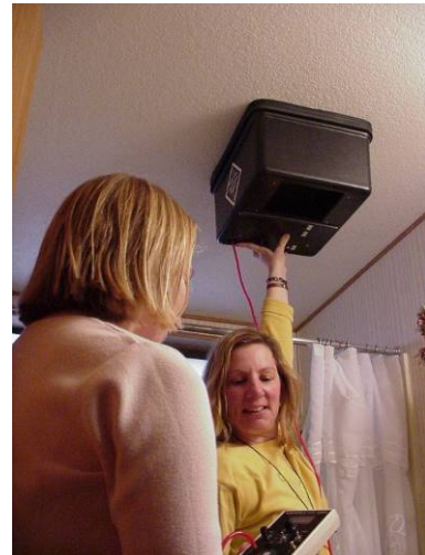
Figure 116-1: Exhaust fan flow meter being used to measure bathroom exhaust fan flow
