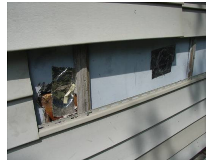
Figure 2142-2: Hole sealed with sheathing tape
