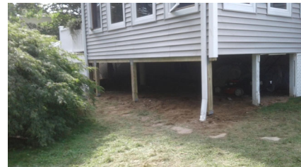
Figure 2154-1: Crawl space supported on piers
