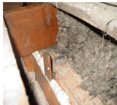
Figure 2122-6: Fur cavity sealed with 2-part spray foam
