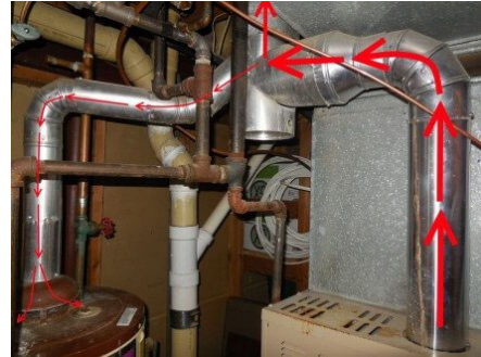
Figure 312-2: Checking for spillage at the water heater after firing the furnace
